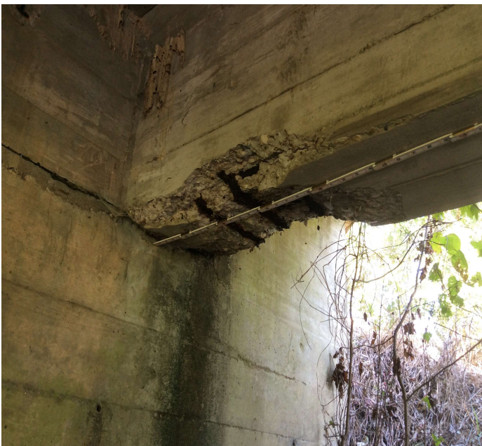
PHOTO 1 Description Span 1, girder 1 at bent 1 Spall with exposed rebar.
